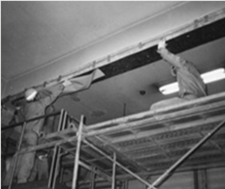
Flexural strengthening
