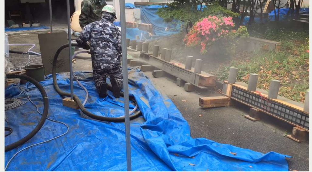
2. Spraying the PCM into the wood frame.
