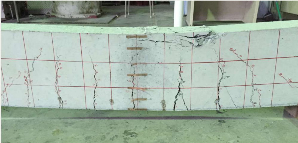
Concrete compressive crushing of [B0]
