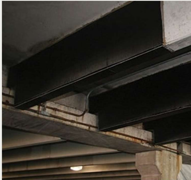
Shear strengthening
