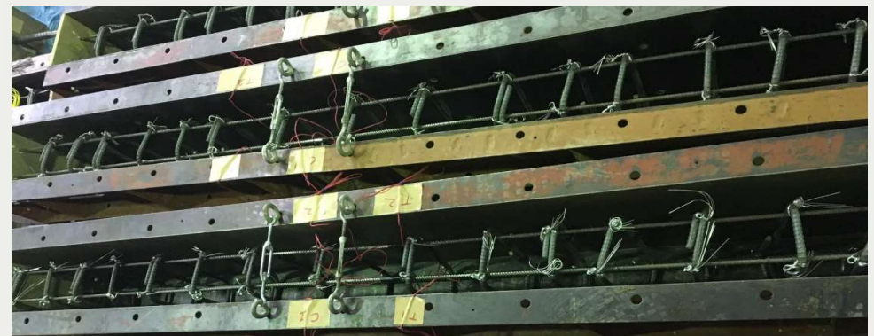
Work frame of RC beams.
