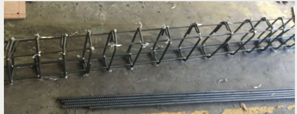
Internal steel reinforcement of RC beams.
