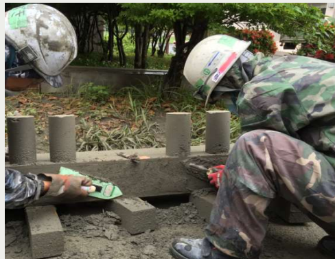
3. Adjusting the final level.
