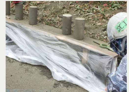
4. Covering with plastic sheets.
