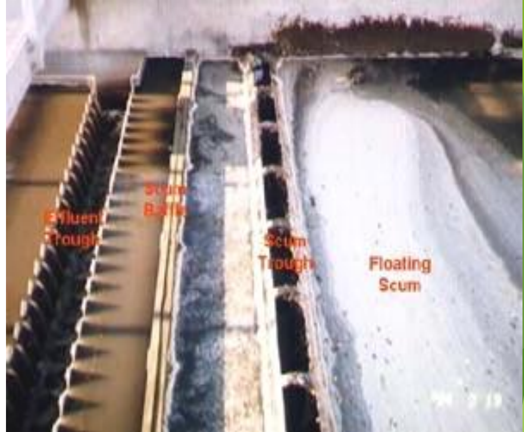
Effluent weir of rectangular sedimentation tank
