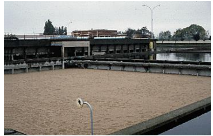
Clean slow sand filter without water layer
